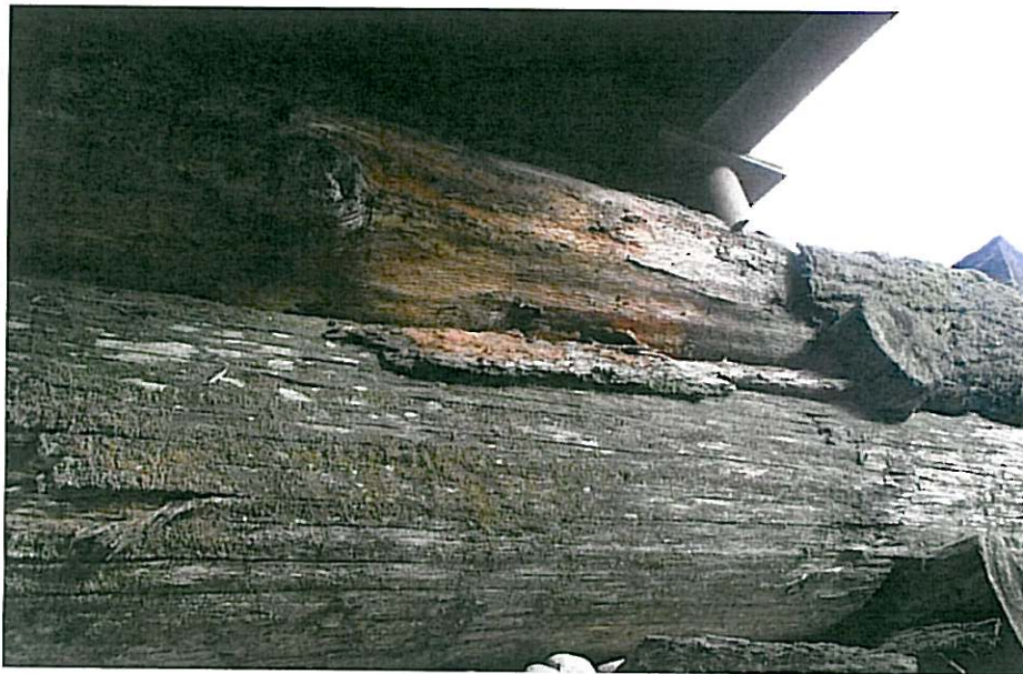
CK-2261 Pier Span 2 (2)
