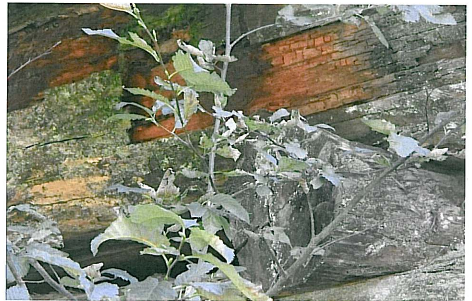
CK-2261 Pier Span 1 Downstream (2)
