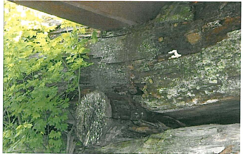
CK-2261 Pier Span 1 Downstream
