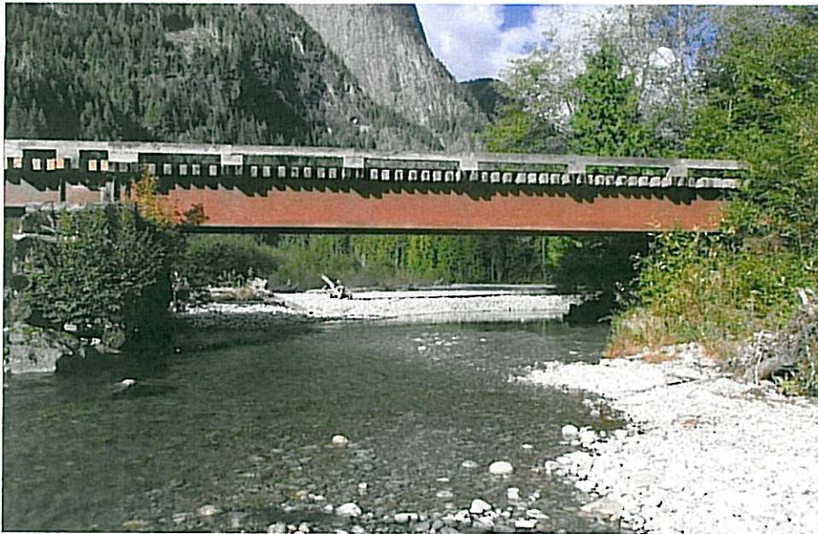
CK-2261 Span 1 Downstream
