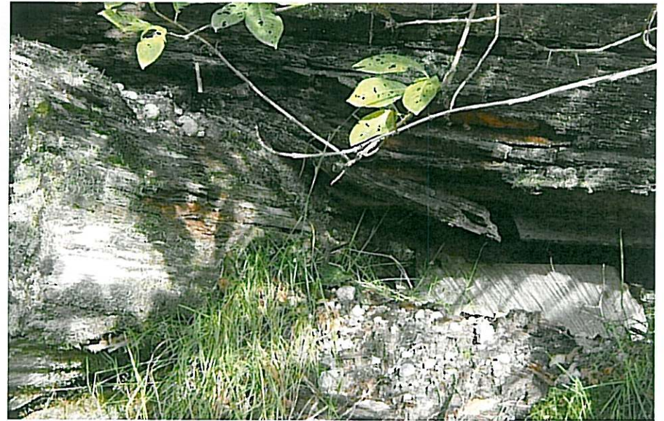
CK-2261 Downstream Left Beam
