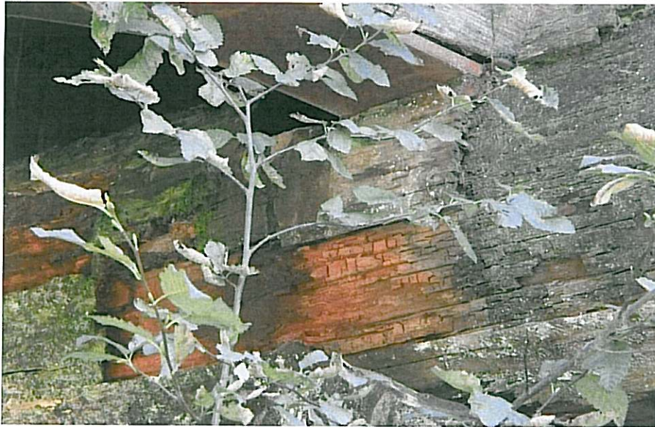
CK-2261 Pier Span 1 Upstream
