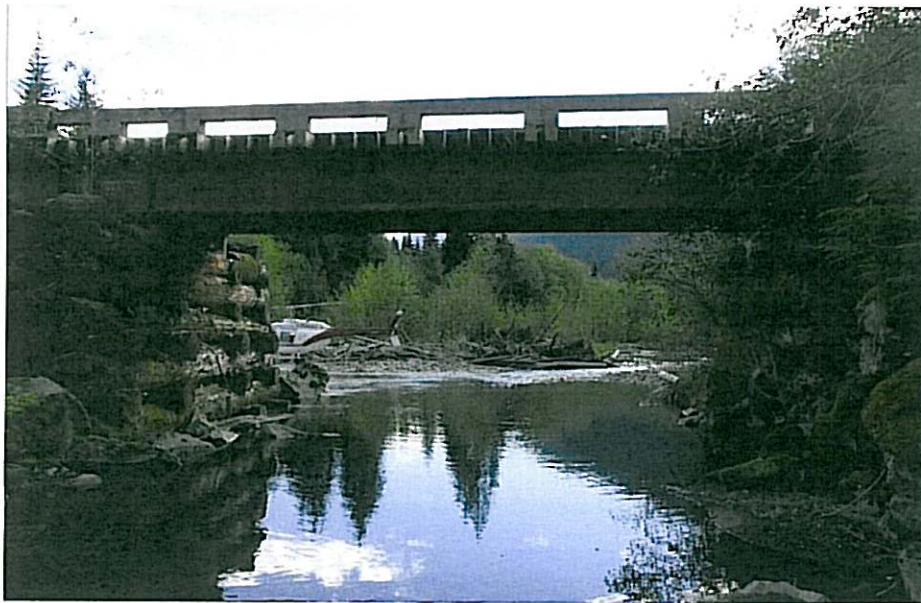
CK-2261 Span 2 Upstream
