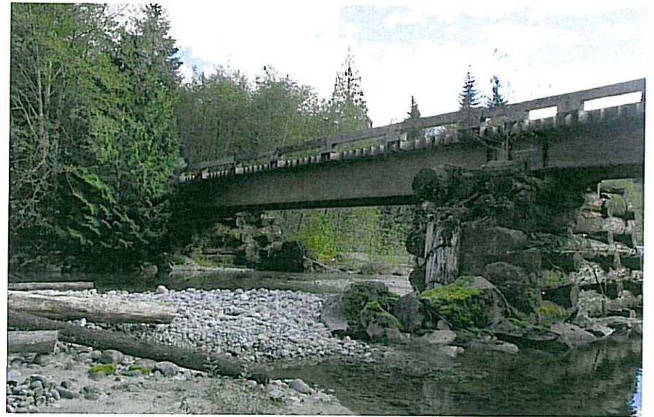
CK-2261 Span 1 Upstream
