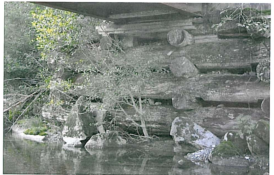
CK-2261 Right Abutment (2)
