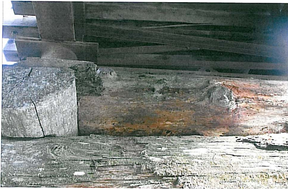
CK-2261 Pier Span 2
