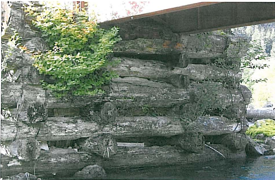
CK-2261 Right Abutment
