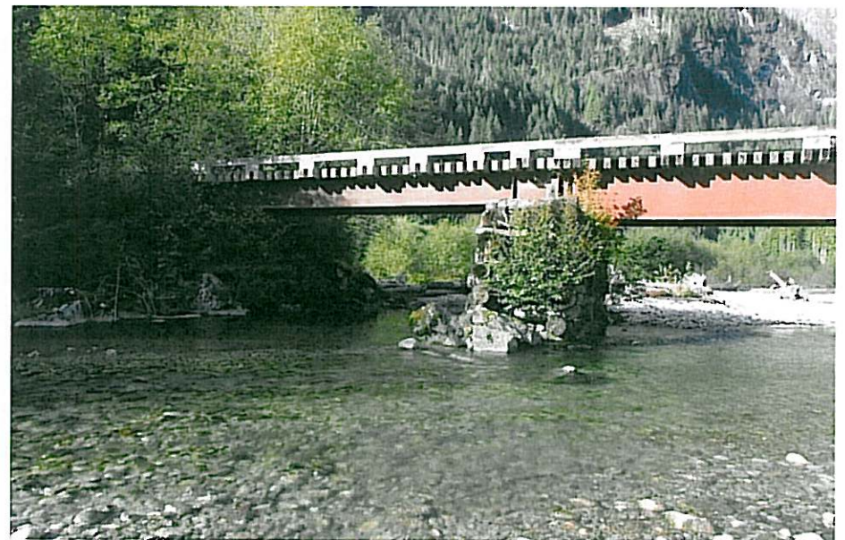
CK-2261 Span 2 Downstream
